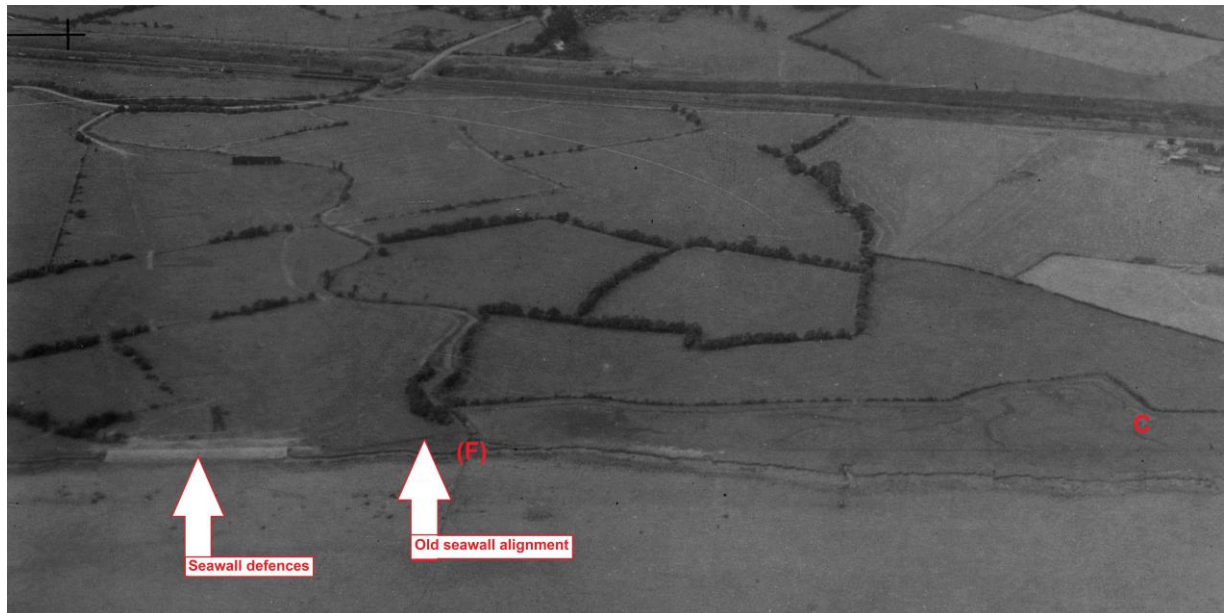
Photograph B: showing 1951 Seawall construction
